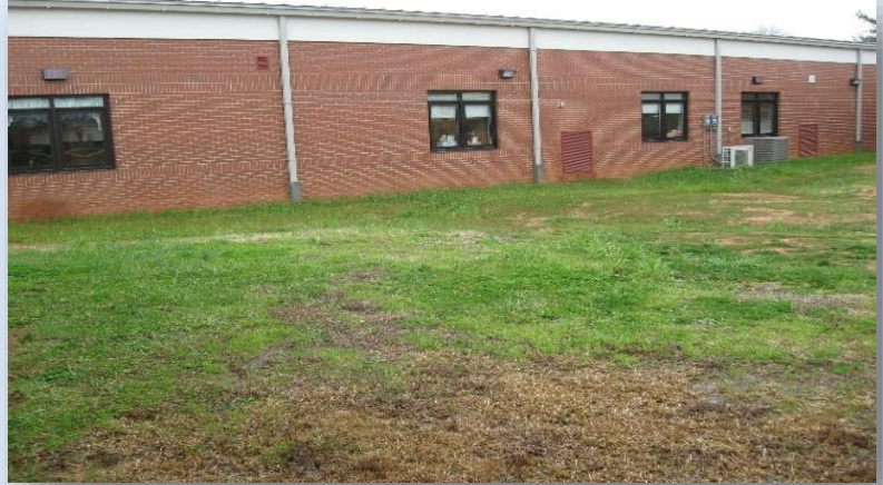
Present condition of our courtyard.
